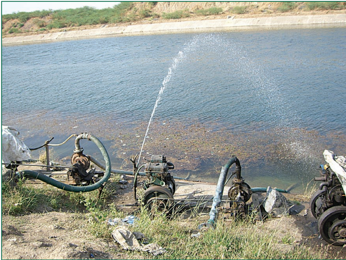
Pumpset drawing water from Sardar Sarovar, main canal, Gujarat
